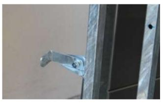
Mount the two door latches as shown. One disc is to be mounted between the stop and the latch. At the rear door, tighten the stop nuts only enough to ensure that the door latches can still be moved easily.
